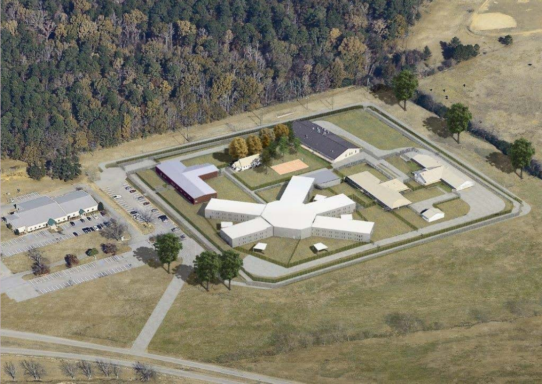
New SVPTP Building Broad River Correctional Institution Campus
